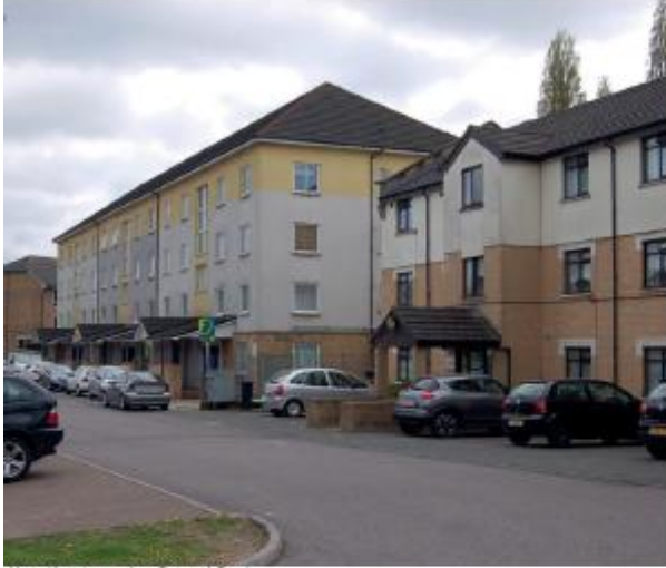
9. Varied housing stock on Denmark Road
